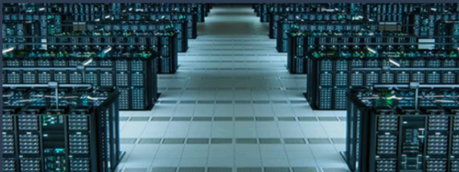
Source: Canada Construct Connect
